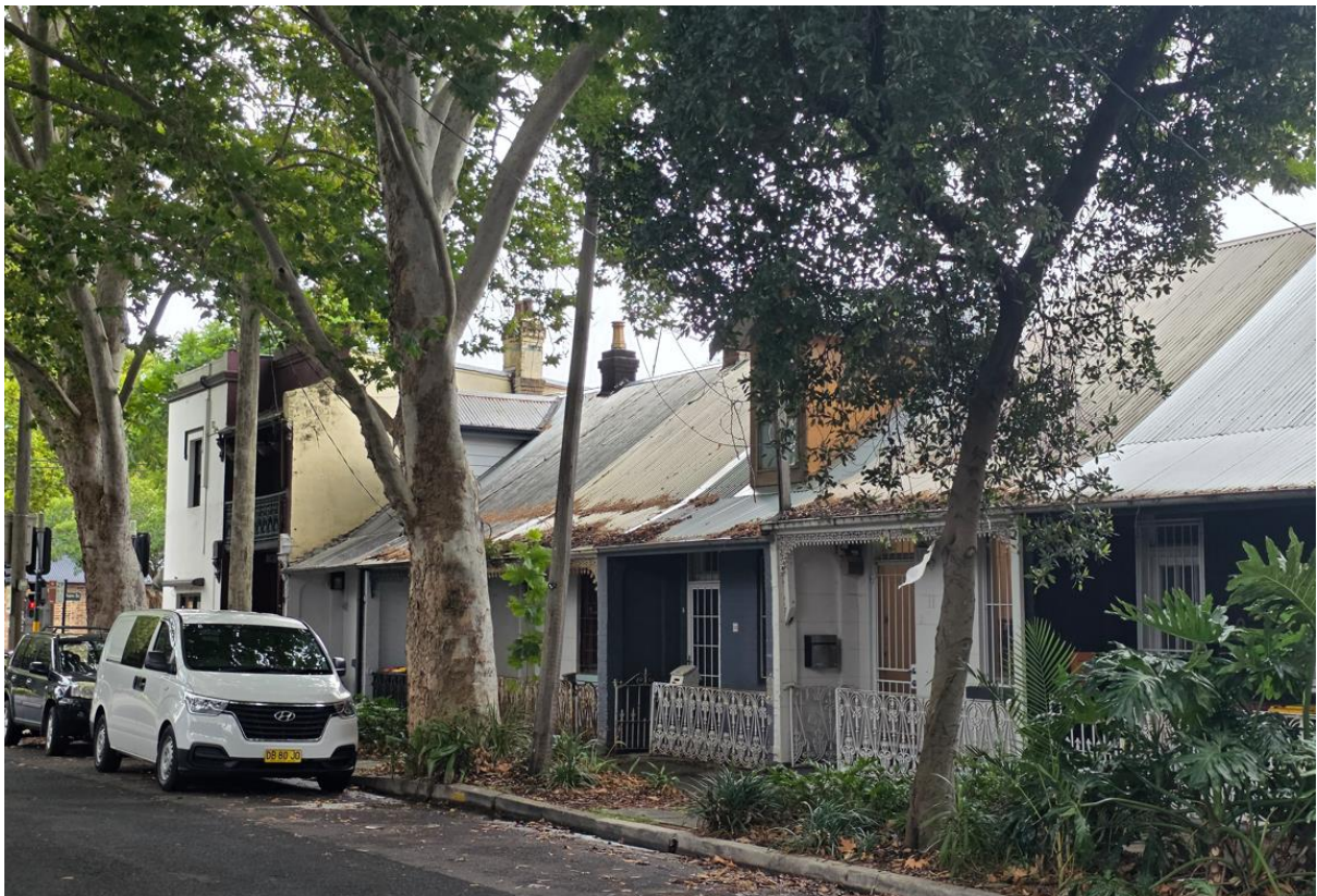
Figure 4: Site (left) viewed from down Buckland Street facing northwest
